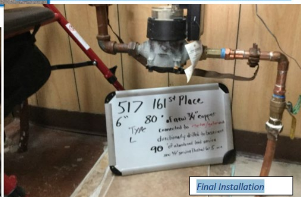
Drilling of Water Service
